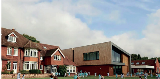
St Andrews School and Halstead School sites
